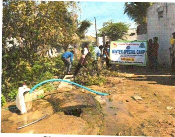
Cleaning near Water Tanks
