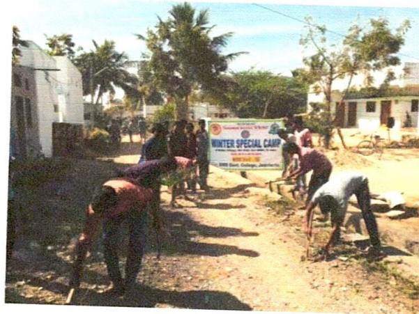
Cleaning the Drainages
