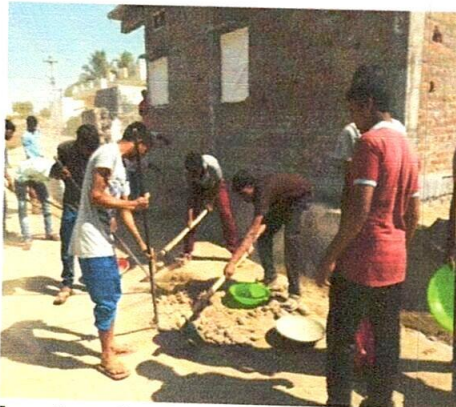
Cleaning the CC roads in the Village
