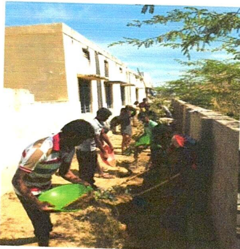
Leveling the School ground with gravel
